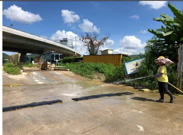
Wastewater treatment facility was properly implemented and bund was installed to prevent wastewater from wheel washing flowing to public area.
