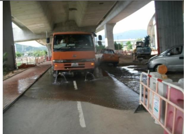
Silt was removed by water tanker.
