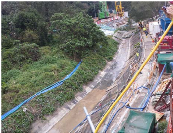
Photo 9 During site inspection on 10 March 2016, it was observed desilting work at upstream portion was completed
