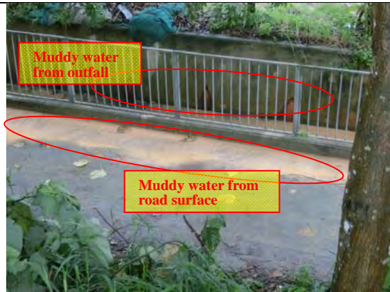
Photo 3 Muddy water was observed flowing from the outfall and public road into the existing channel. The source of muddy water is unknown as it is located outside site boundary.
