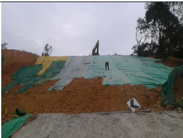
Photo 5 Covering of the open slope to minimize muddy runoff was in progress on 5 February 2016
