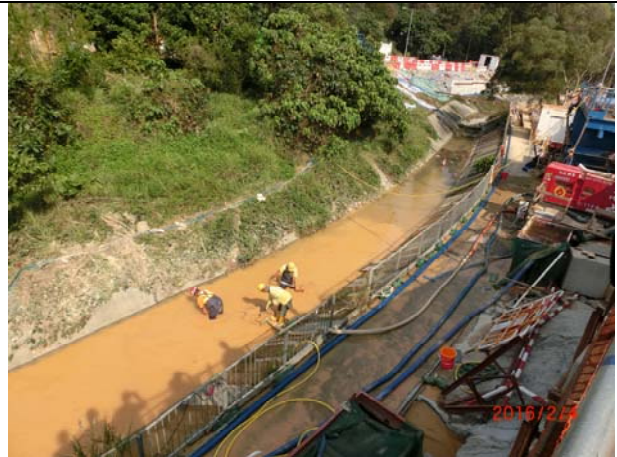
Photo 4 Run off from excavation area was flowing into the existing channel during rainstorm. (4 February 2016)
